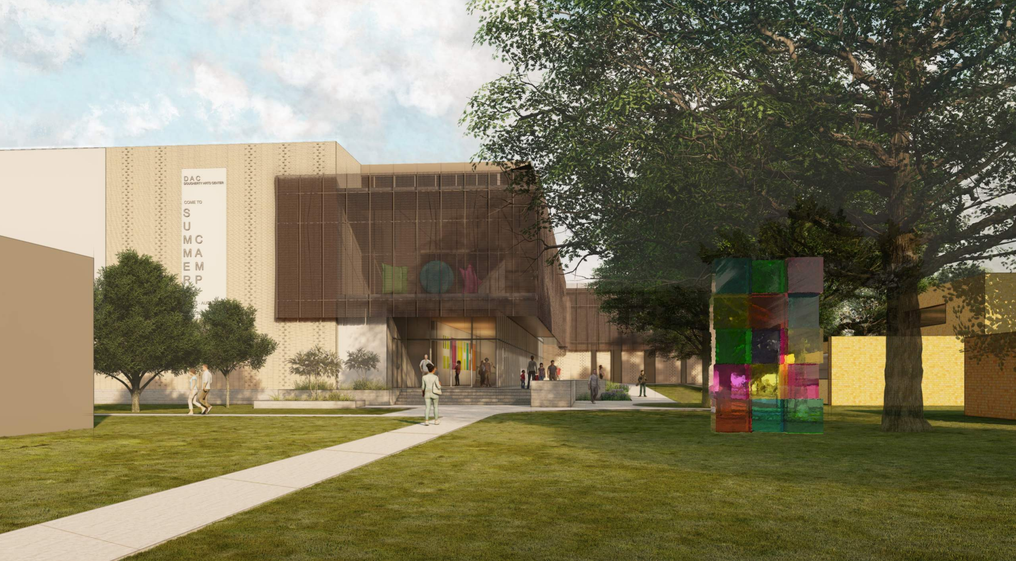
VIEW FROM ZACH, LOOKING WEST
